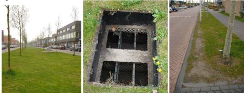
Fig. 3. Left: a wadi. Centre: Infiltration trench underneath the surface of the wadi. Right: Small stormwater infiltration area with compacted soil due to car parking.
