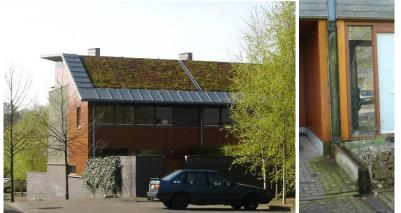
Fig. 19. Left: Green roof with zinc edges. Right: Visibility of stormwater and zinc 'down-pipe'.
